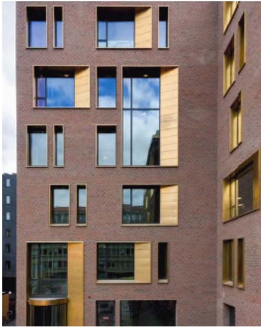
Image 4: Visual showing use of colours and materials and a precedent using brick and bronze cladding
